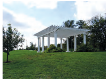
Shoal Creek Parkway north of 85th Terrace looking southwest
