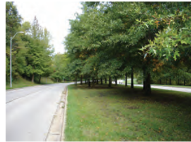
Searcy Creek Parkway looking north
