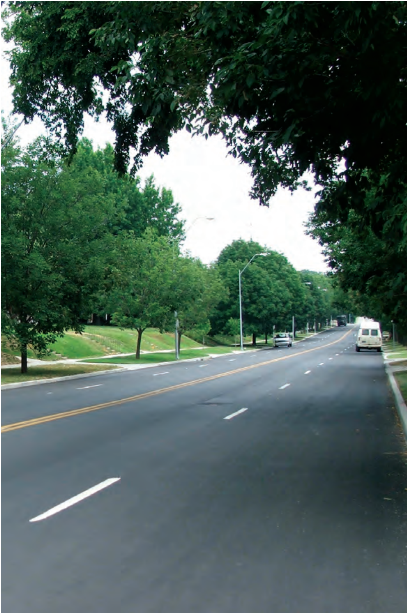
Gregory Boulevard just east of Holmes Road
