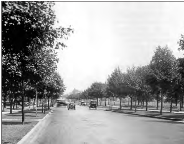
Benton Boulevard, north from near Thirteenth Street, 1910s
