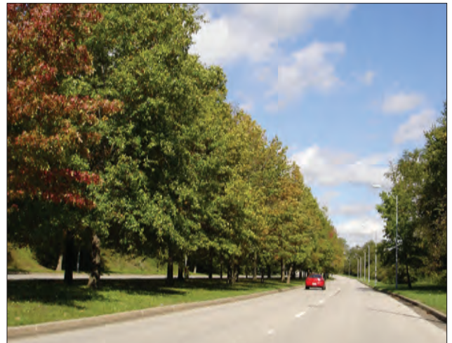
Searcy Creek Parkway looking north
