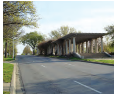
Looking north from 11th Street and southbound The Paseo
