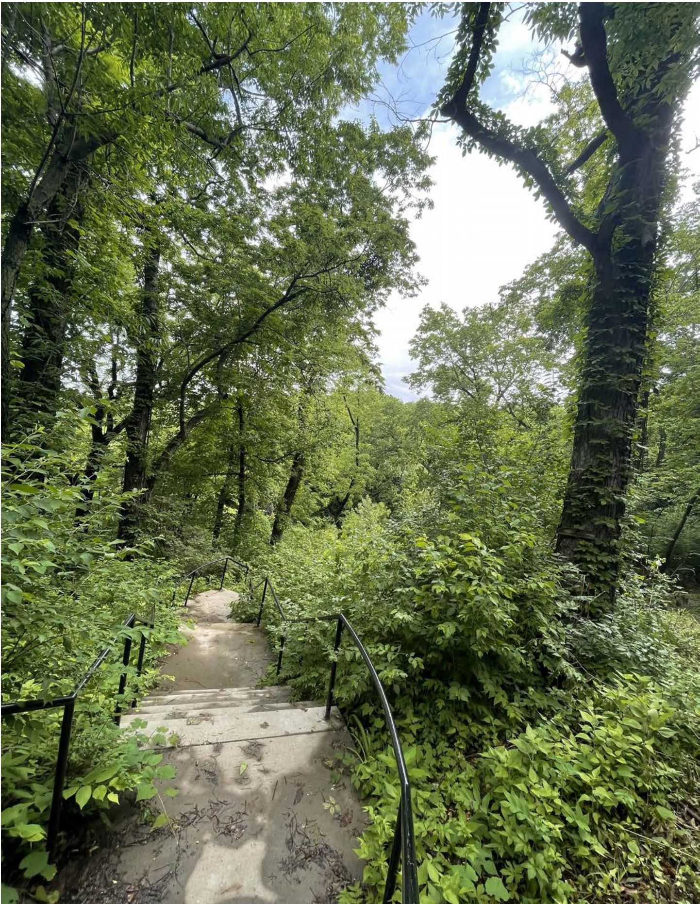
Stair behind Colonnade at Concourse Park
