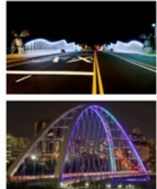
MLK PEDESTRIAN BRIDGE
