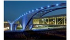
MLK PEDESTRIAN BRIDGE
