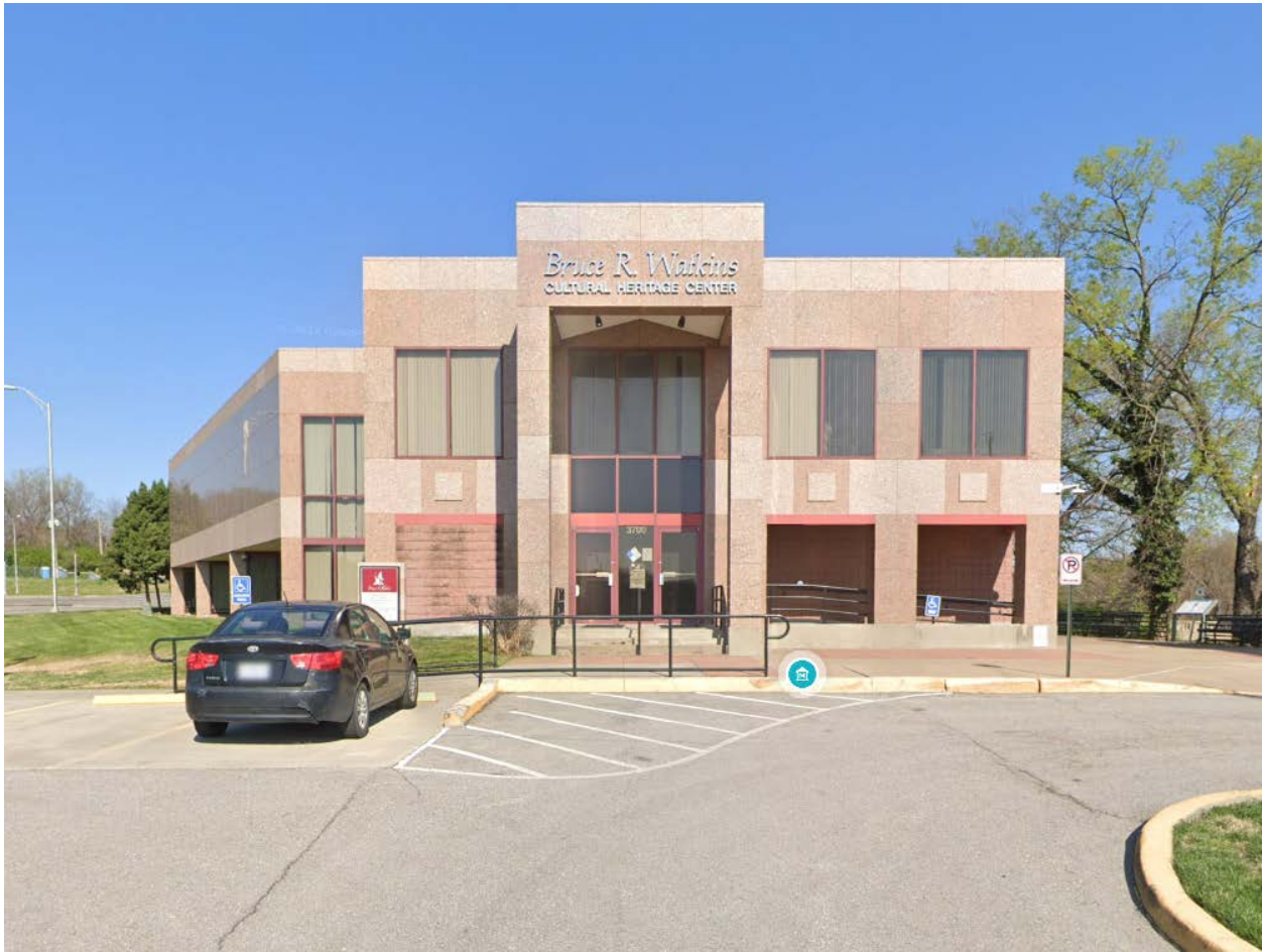
Figure 2 Exterior Photographs Bruce R. Watkins Cultural Heritage Center & Museum
