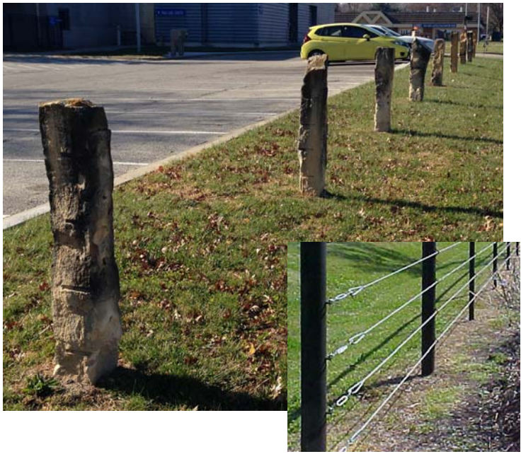
LIMESTONE COLUMN FENCE WITH WIRE CABLE RAILING
