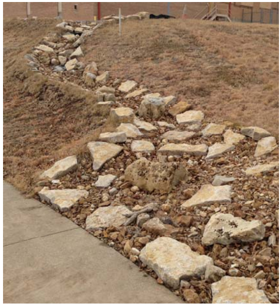
ROCK LINED DRAINAGE SWALE
