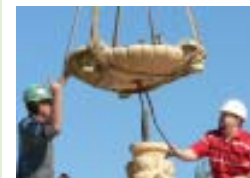
october 1 Meyer Circle Sea Horse Fountain Repairs Begin
