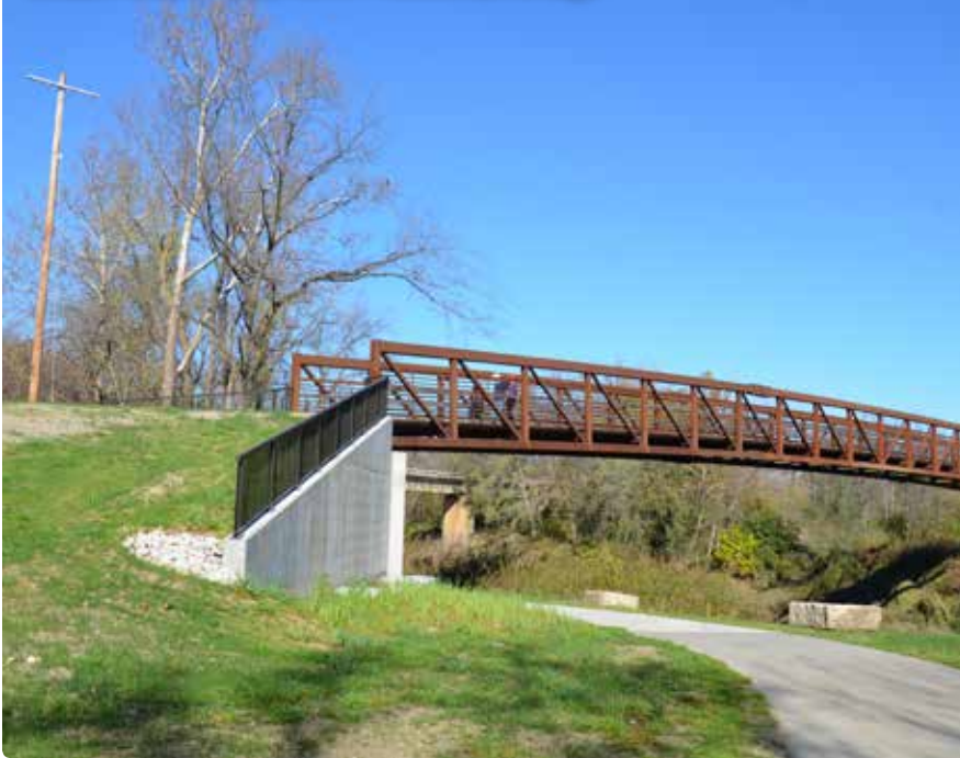
Indian Creek - Blue River Pedestrian Bridge
